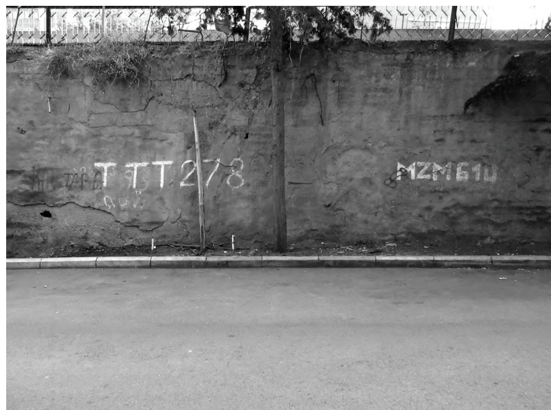
Informal claims to parking in a Saburtalo neighbourhood by indicating license plate numbers on the wall
